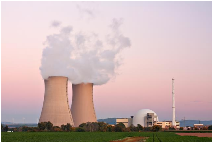
Grohnde/Lower Saxony nuclear power plant
